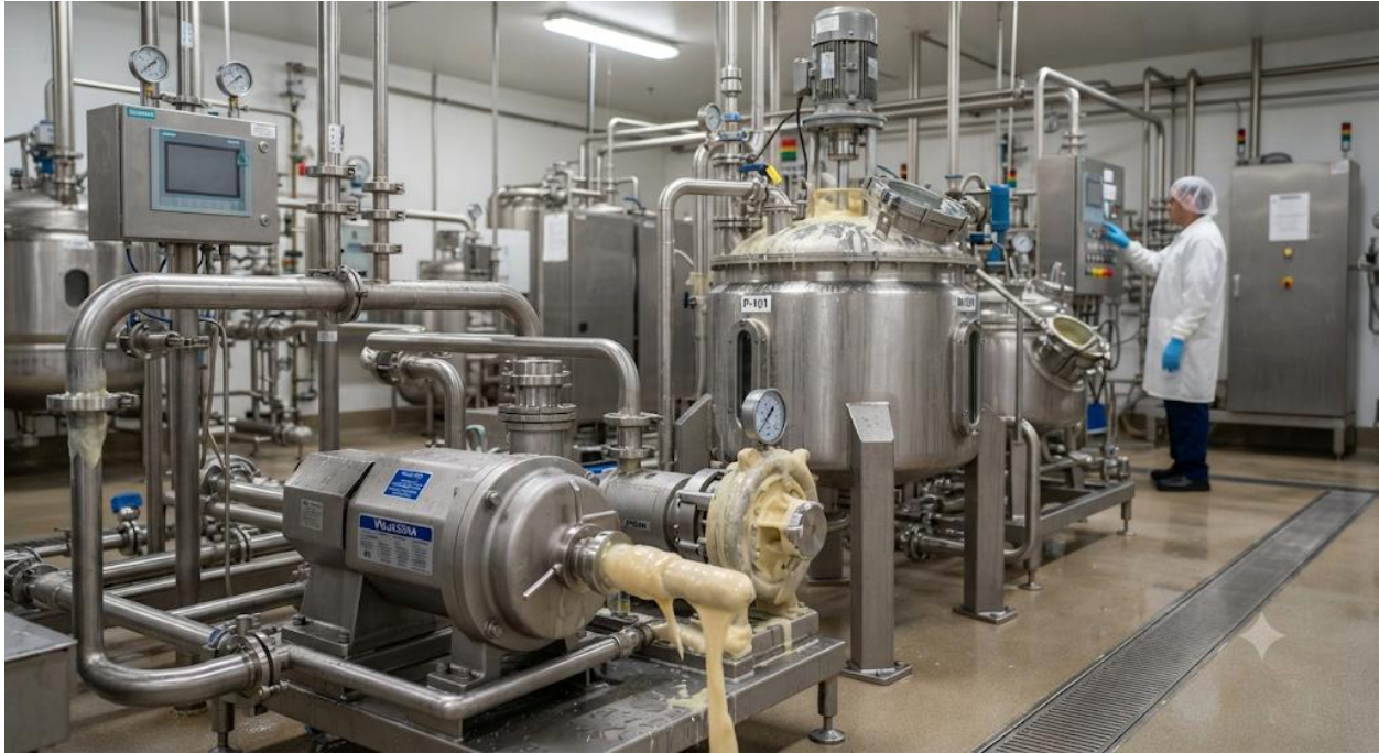
Image of industrial pumps and mixers used in food processing Plate 3.2: Pumps and mixers in food engineering
