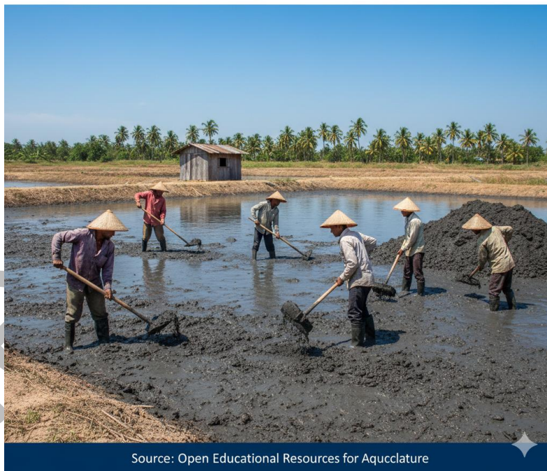
Plate 5.1 Cleaning and Desilting Ponds
