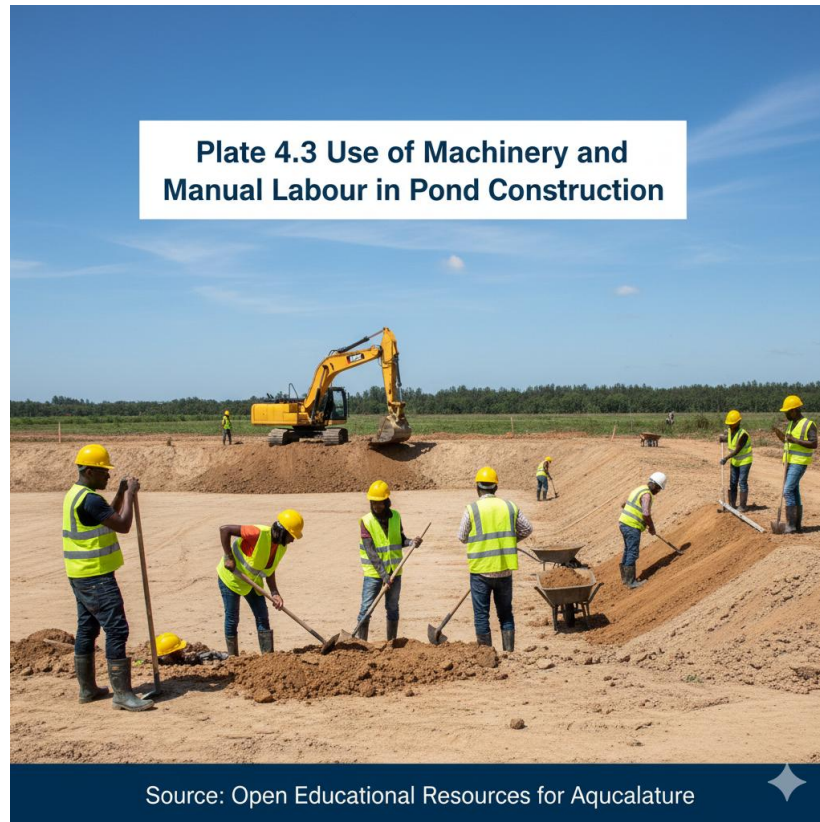
Plate 4.3 Use of machinery and manual labour in pond construction
