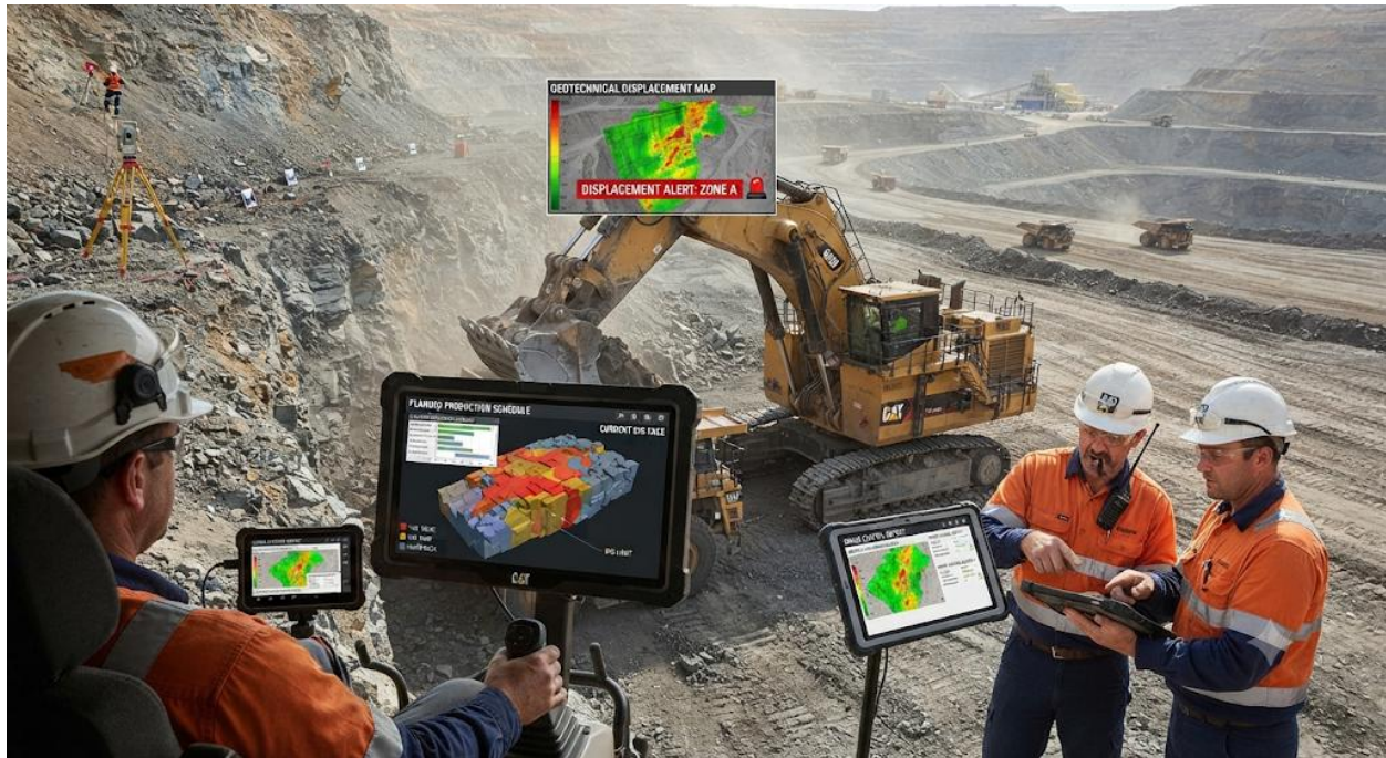
Photograph of excavation operations guided by reserve estimation data. Plate 4.4: Excavation and production scheduling supported by survey data
