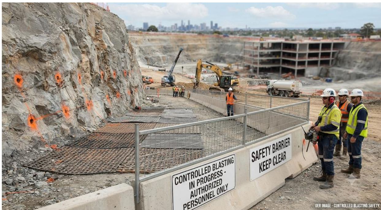
Image showing controlled blasting near a construction site Caption: Plate 4.1 Controlled blasting in construction projects
