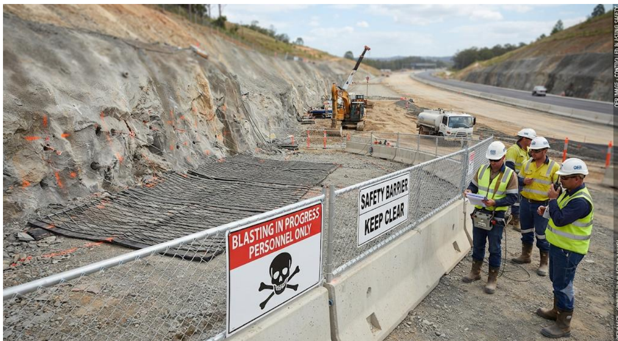
Image showing blasting in a road construction project Caption: Plate 5.1 Controlled blasting in road construction
