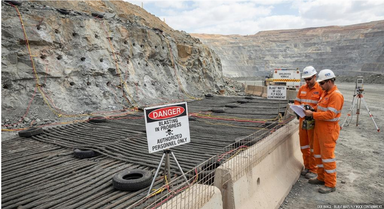
Image showing blast mats covering a blast site Caption: Plate 5.3 Blast mats used to contain fly rock
