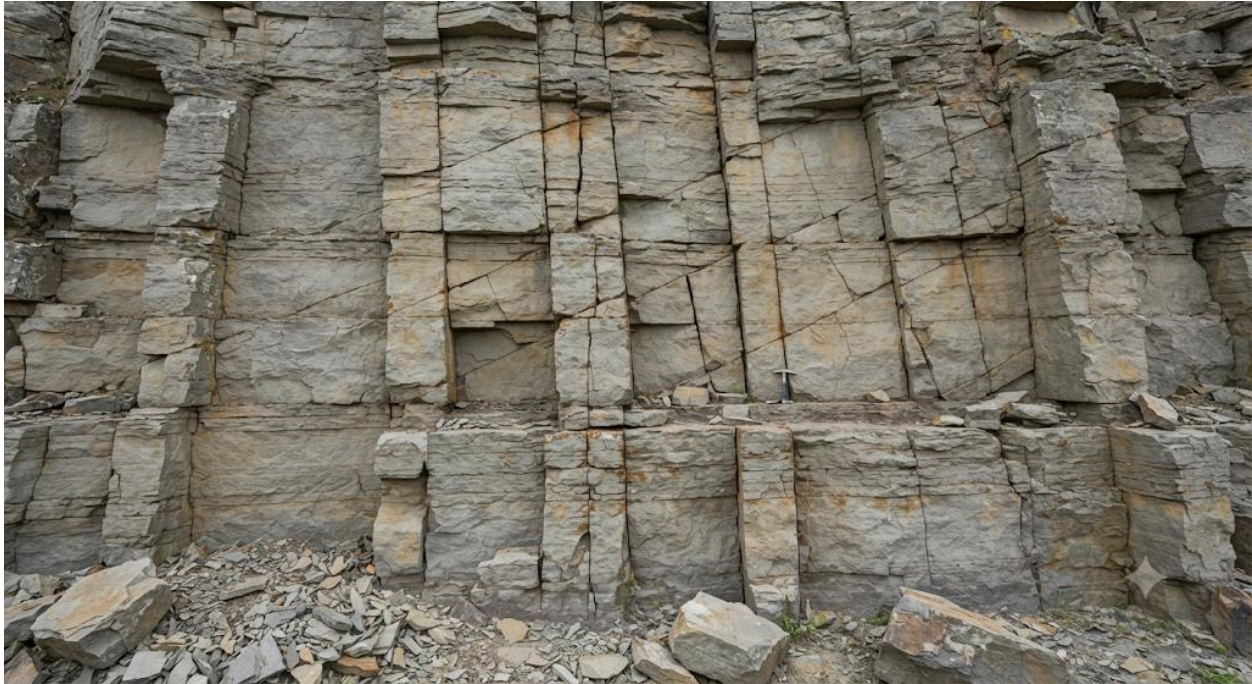
Photograph of jointed rock surfaces in a cliff face. Plate 3.2: Joints in rock formations
