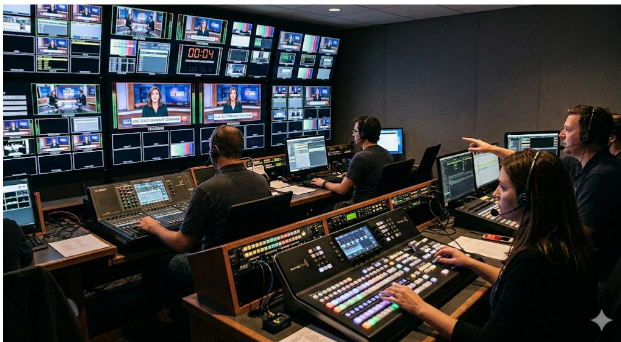
Image showing a television control room with staff at work Plate 1.2 Control room operations in a broadcast station
