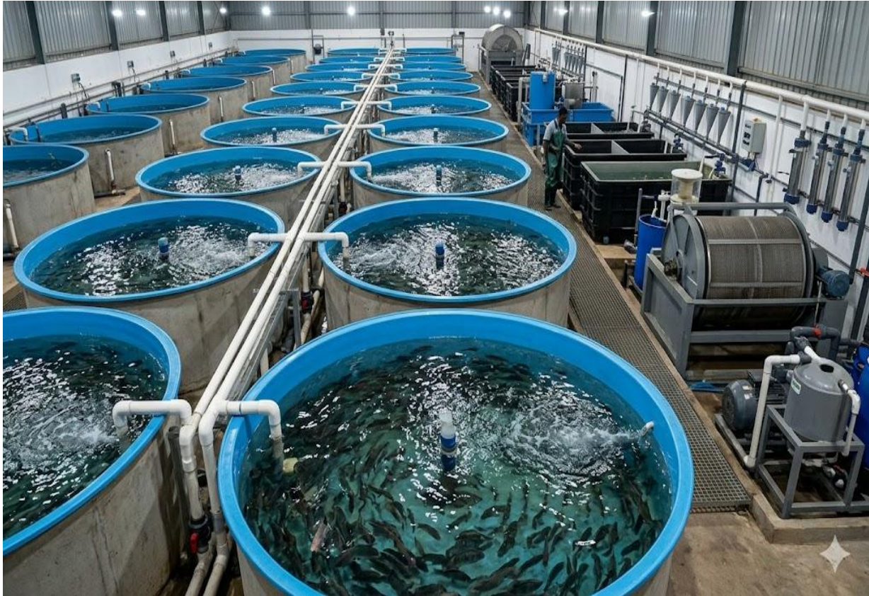
Plate 1.1: Interior of an intensive fish hatchery showing recirculating aquaculture system tanks and associated water treatment equipment
